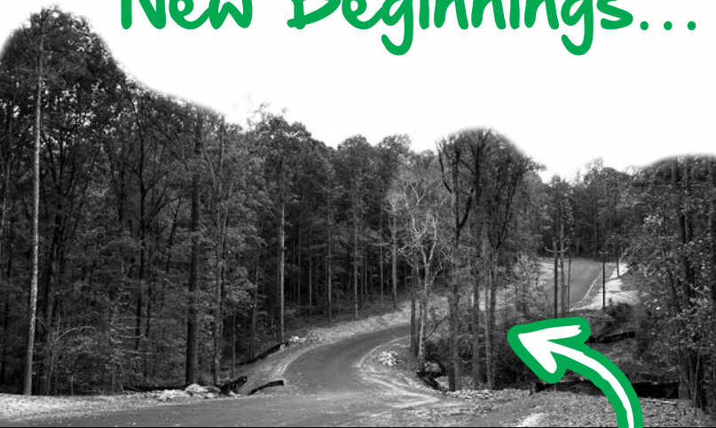
New road to our Barn Center and Processing Area
